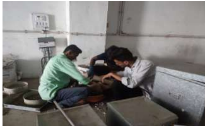
Figure No.1 (Mixing of Concrete)
